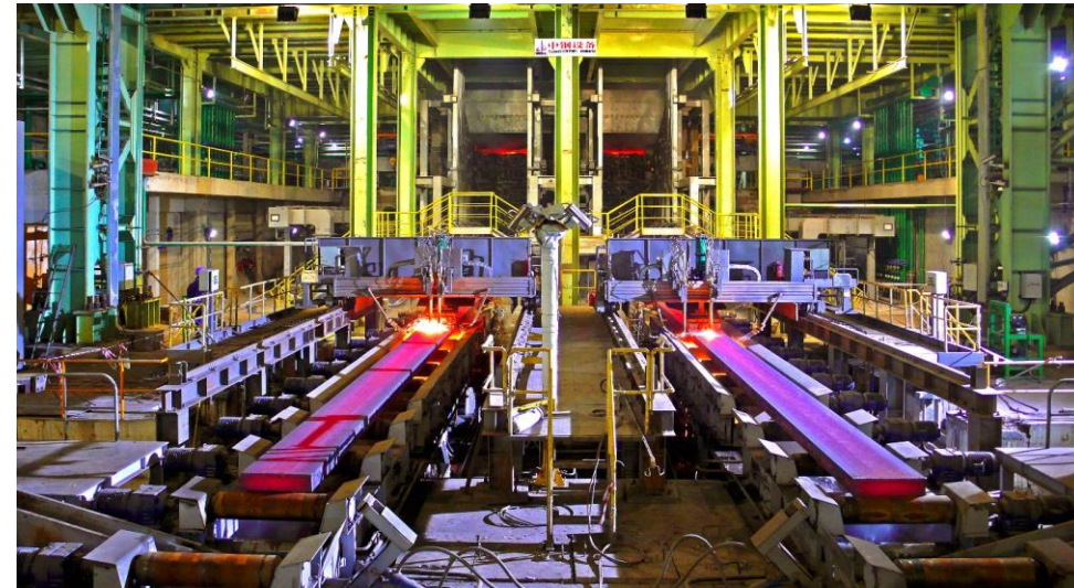
Tosyali Continuous Slab Caster Project, Turkey
